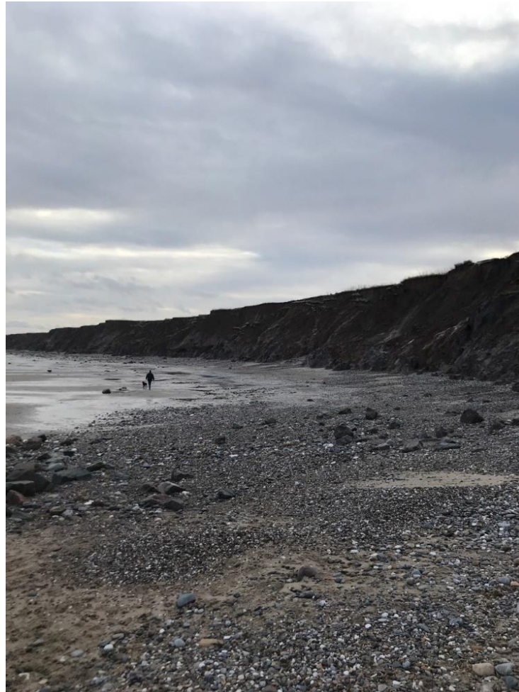
Plate 1: High, unstable cliffs within the C2x landfall zone.
