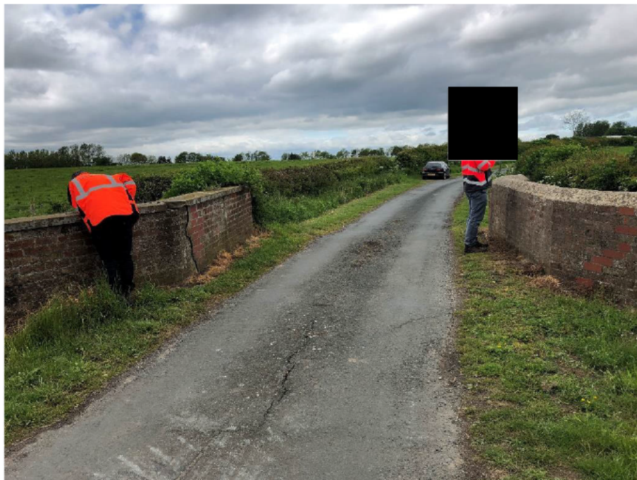
Plate 2: Existing Bridge across The Earl's Dyke.
